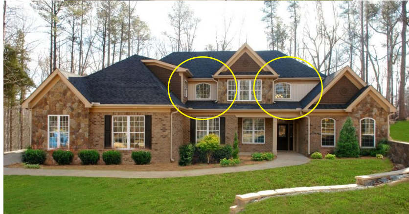
Figure J: Two images of the acceptable use of vinyl as trim in circled areas
