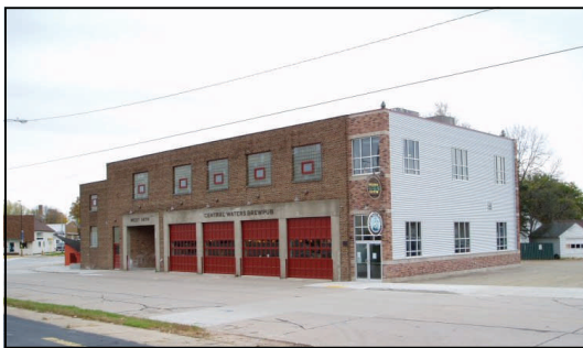
After Photo: Renovated Building Exterior
