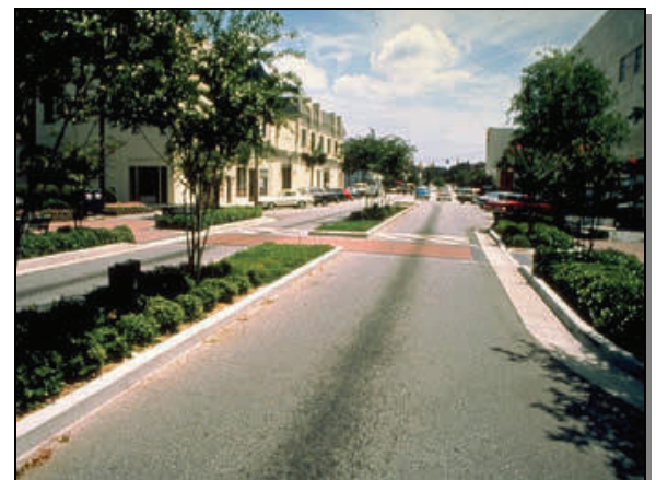
Landscaped median island and textured crosswalk
